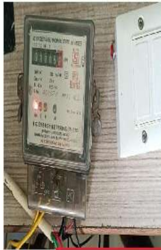
Compressor cut off device connected with sub-meter for testing
