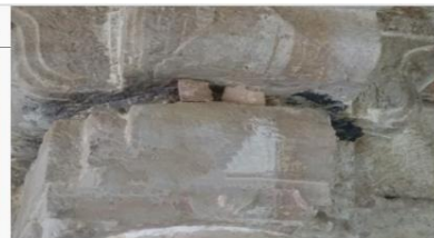
Fig No. 37 Picture showing Minor gap in outer portion of pillar
