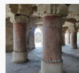
Fig No. 38 Picture showing presence of Iron Oxide of pillar
