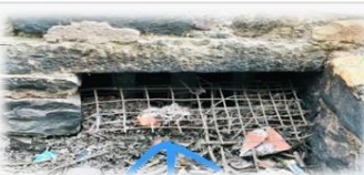
Fig No. 19 Choked Drainage
